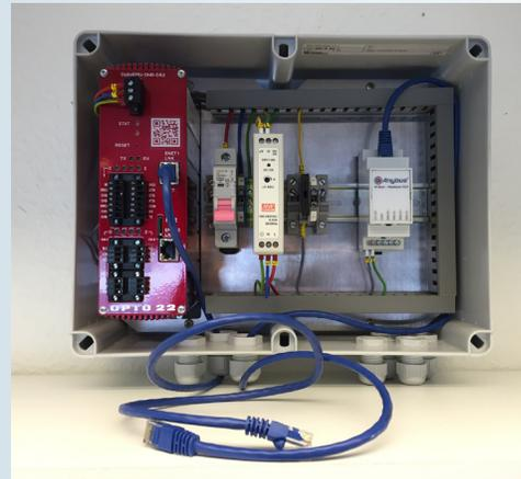
The Opto 22 controller to the left and the Anybus M-Bus to Modbus-TCP gateway to the right.
